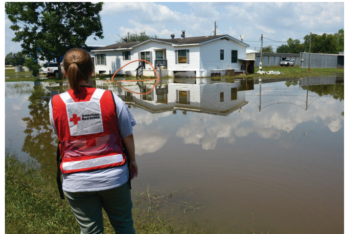
A Red Cross worker assesses damage and standing water levels in Wharton, Texas, nine days after Hurricane Harvey made landfall. Photo: Daniel Cima/American Red Cross
